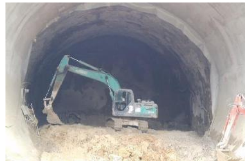
Fig.2 Drilling rig platform site preparation
