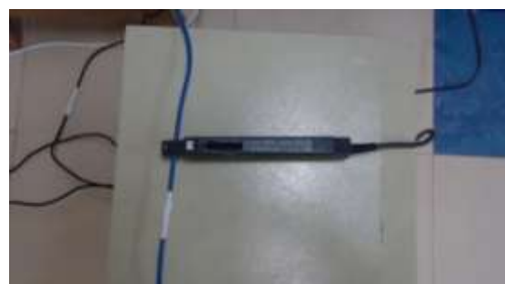
Figure 15 Current probe clamped on phase wire
