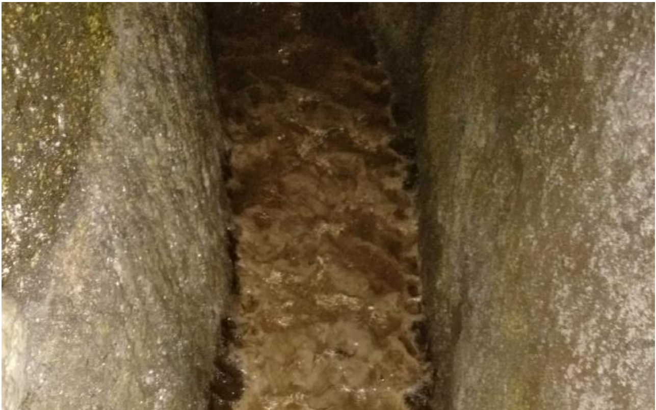
Fig. 3 – Photographic shots inside the ancient and underground conduit. Credits: Giancarlo Valle; Arco di Diana APS.
