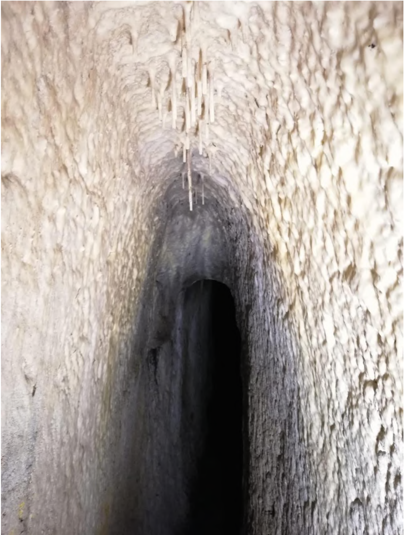
Fig. 21 – Presence of calcium carbonate statallites inside the ancient tunnel explored on 9 September 2021. Giancarlo Valle, Credits: Arco di Diana APS.
